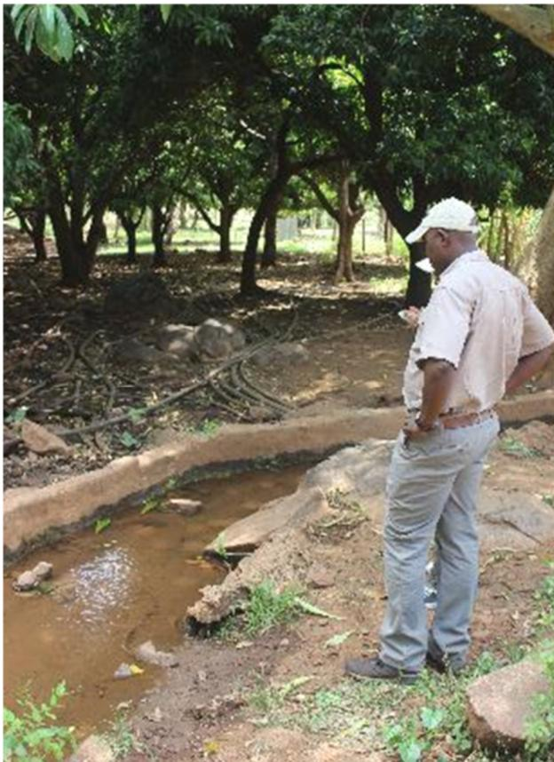
A gravitational system from the waterfalls in Lepelle are used for irrigation, bathing and drinking. According to Patricia, this system was initiated in the 1960's
