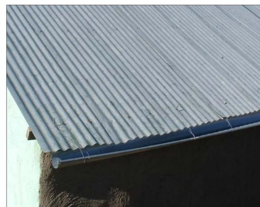
*Figure 4.15: Sheet metal gutter fixed to roof sheets with 3mm fencing wire*
