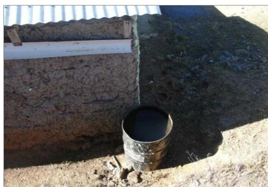
There are three main components to roofwater harvesting; the **roof**, the **gutter** and the **storage tank**. What follows is a summary of each of these components, and practical suggestions as to how each can best be utilised.
