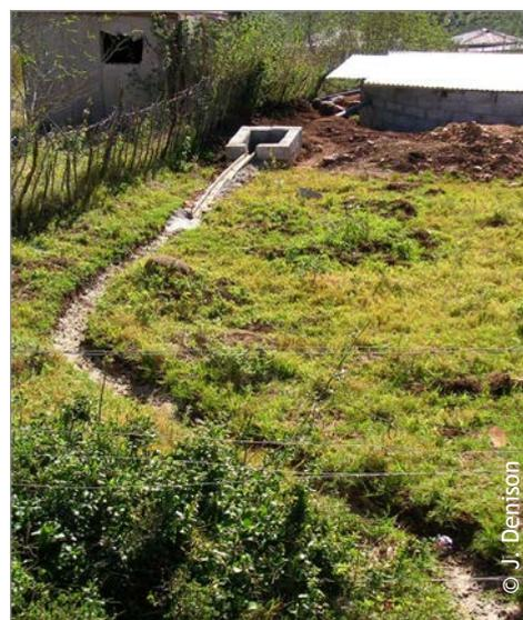
Figure 4.1 Diversion furrow leading to a catchpit
