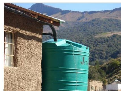
*Figure 4.16: U-Round guttering used in Cata Village, Eastern Cape*
